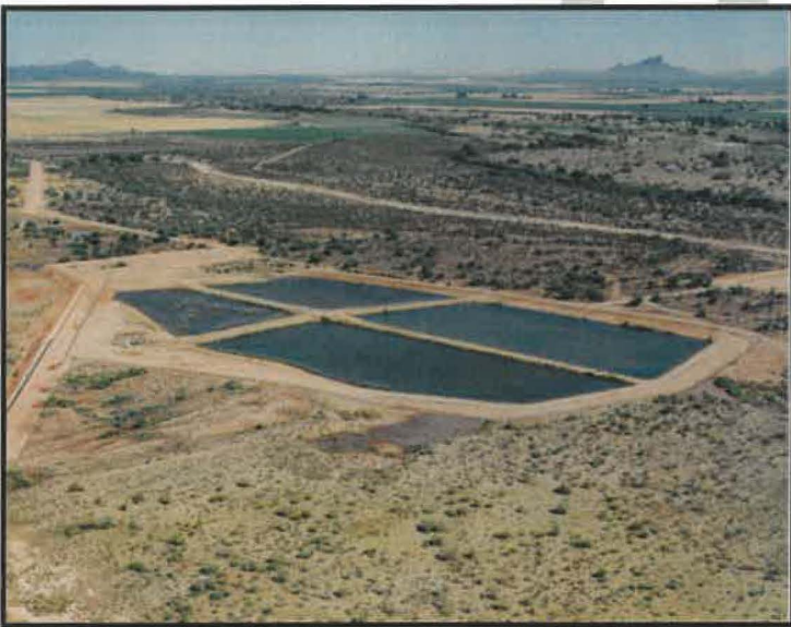
Avra Valley Recharge Project
